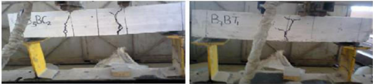
Fig. 2- Flexural failure of beam with circular and triangular bamboo as reinforcement
